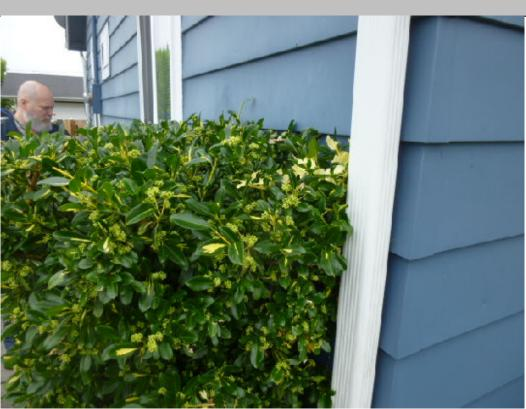
Grounds appear to be maintained. Vegetation was found to be contacting the exterior of the home. Recommend trimming vegetation away from structure to increase ventilation and sunlight and reduce moisture problems.
