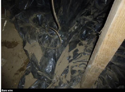
The following type of branch wiring was found throughout the structure: Copper wire, The following wire system is present: Romex, All visible wiring appears functional. Bare wires are noted in crawlspace under house. Wires need to be secured in junction box. Have a licensed electrician make further evaluation and corrections as needed.
