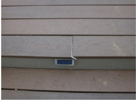
The decking boards appeared functional and without rot conditions. Lag bolts were present securing the deck's header joist to the exterior wall. Flashing was found to be installed above the header joist where the deck is attached to the home. Deck board at rear step has shifted and needs repairs. Consider replacing board as needed.
